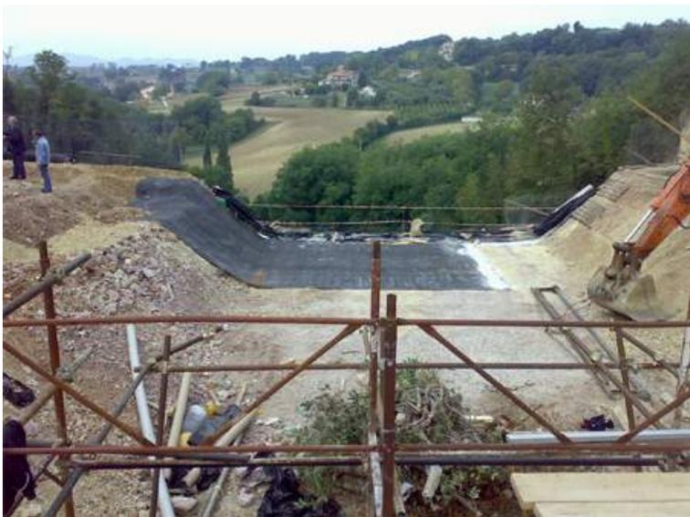
**Figure 8.** Section of “Fosso della Rocca” stream in the stilling basin. GCL installation
