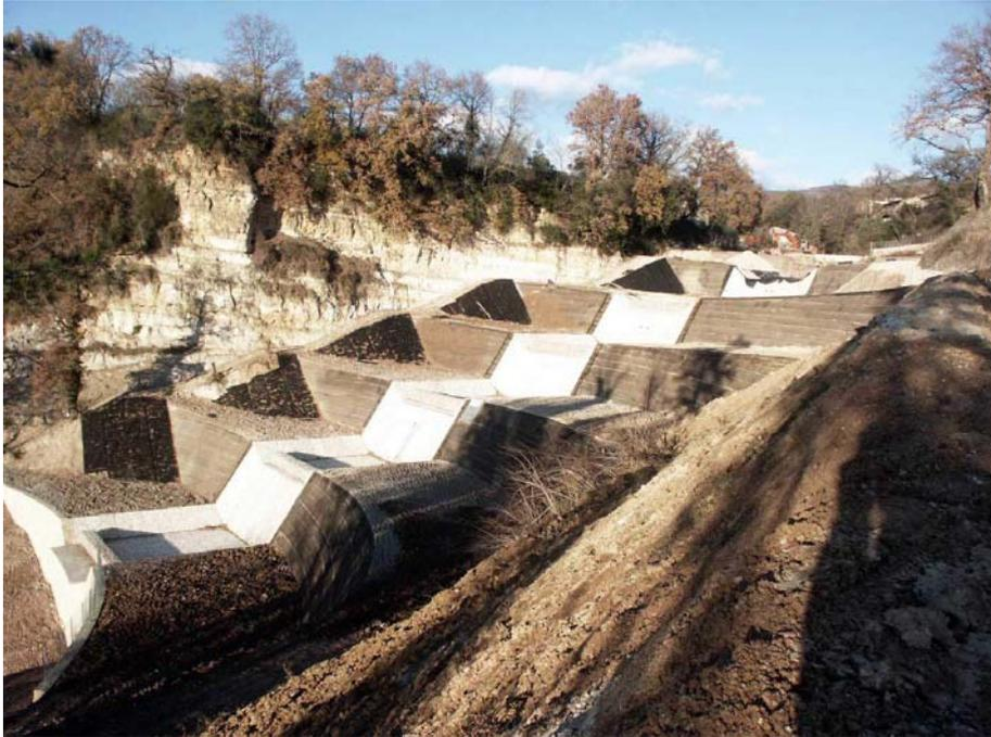
**Figure 9.** Overall view. Reinforced slopes, central water chute and erosion control geomats on the peripheral slopes
