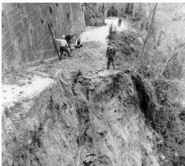
**Figure 1.** Landslide at the toe of the retaining wall bordering the village
