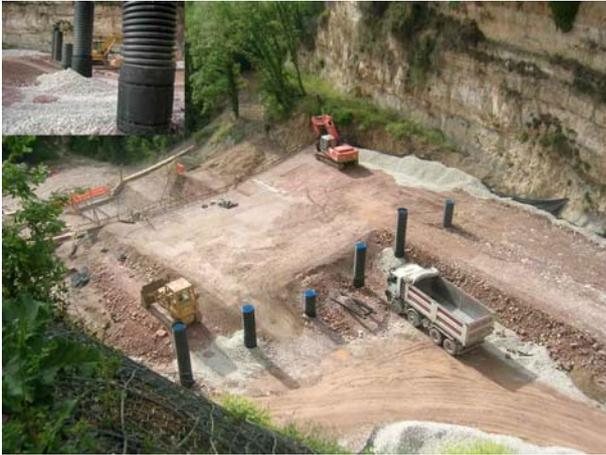
Figure 5. Vertical pipes interconnecting horizontal drainage blankets, both covered with a woven filter
